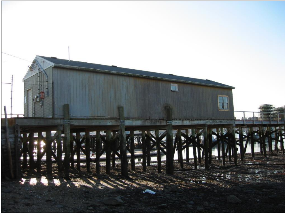
Building at Portland Street Pier – East side
